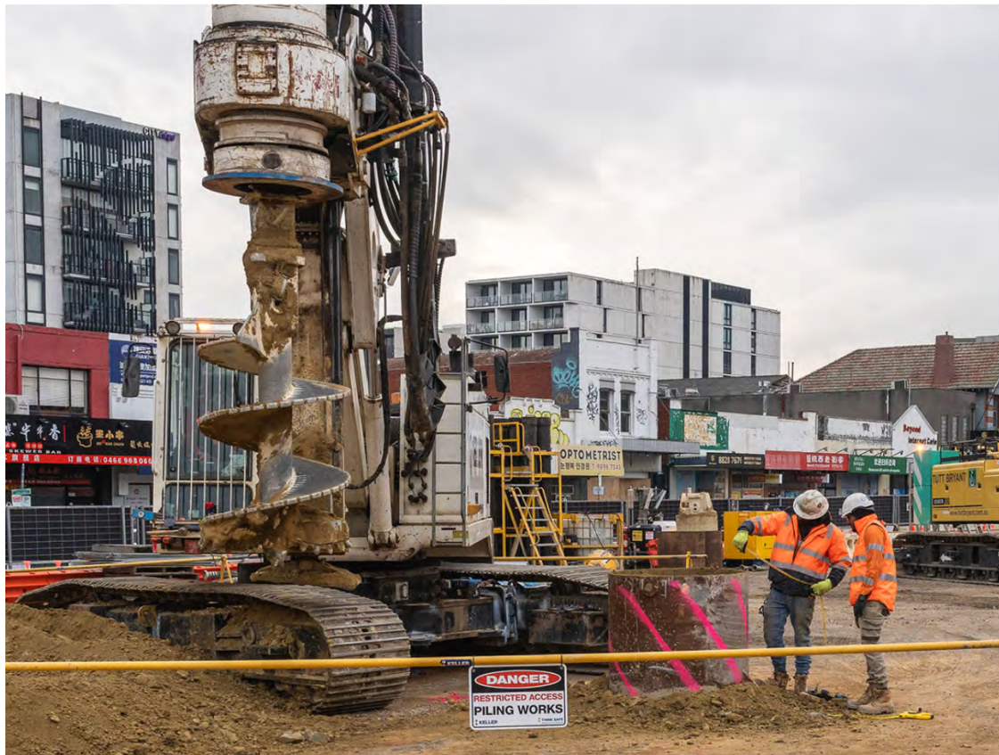
Figure 3: Example of pile driving equipment used in the construction works [2].
