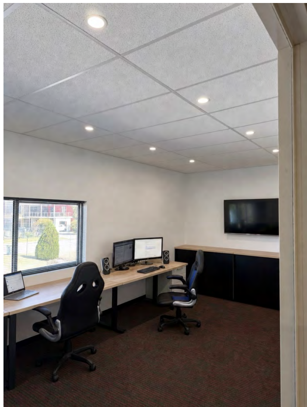
Figure 1: Acoustic tiles absorb some of the noise.
